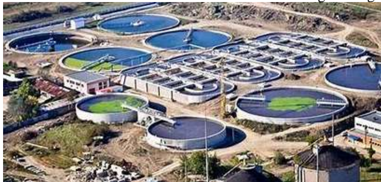
SEWAGE TREATMENT PLANT Source: Louksengineering.com
